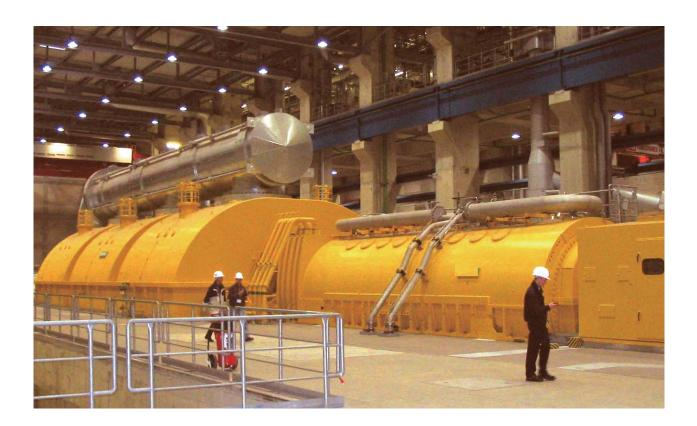
The Turbo-Generator Package consists of a generator, an exciter and a cooler as the packaged operating unit. These 3-phase synchronous turbo-generator packages match with their respective steam turbine units in power. For example, the model number BW-CG-50 package (50 MW) would be used in conjunction with the model number SC-RT-50 steam turbine (50 MW) for a 50 MW power plant.
